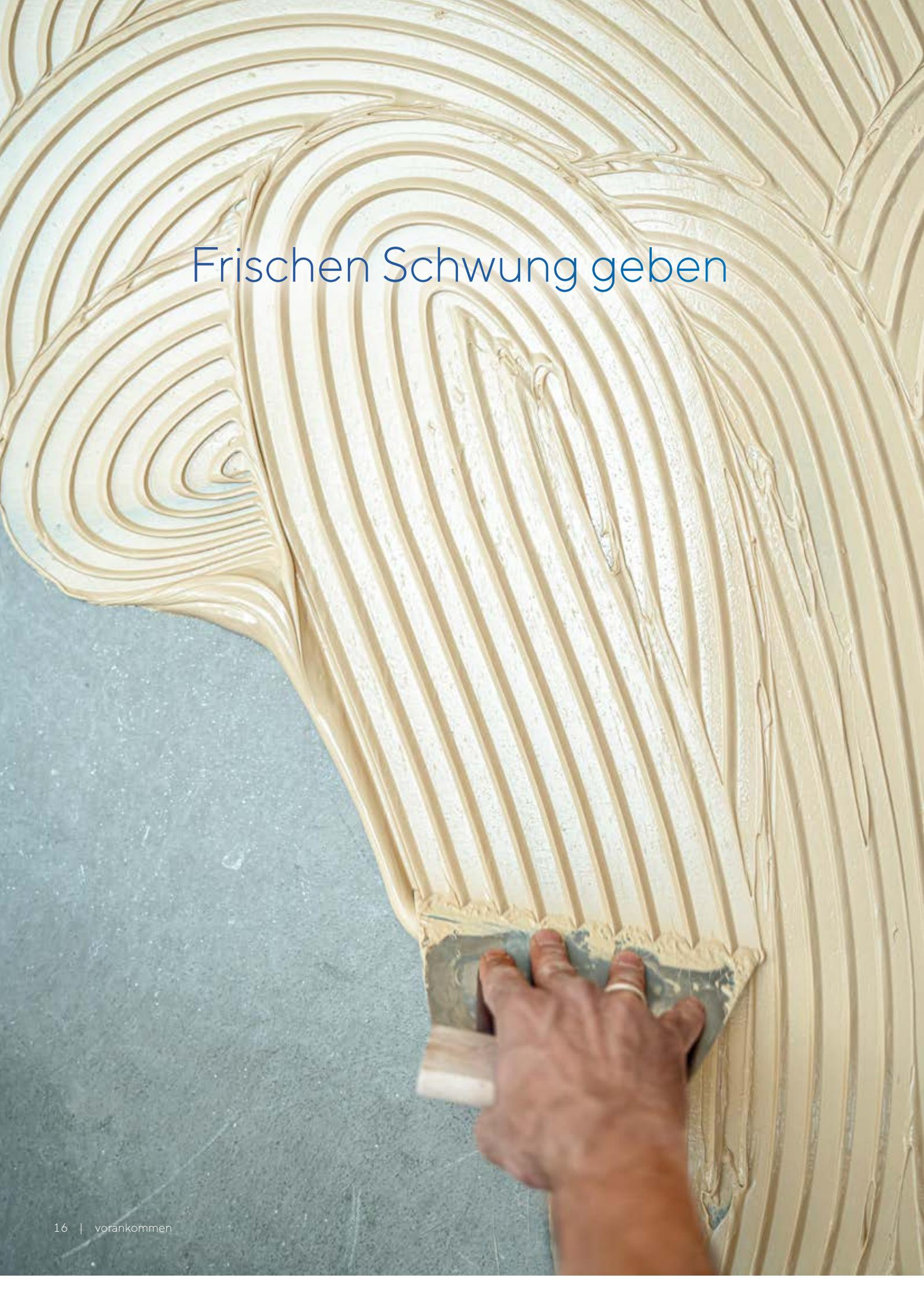
A close-up photograph showing a hand holding a metal trowel with a wooden handle, applying a thick, light-colored plaster or mortar to a wall. The plaster is being smoothed and textured, creating a series of concentric, wavy lines that radiate from the center. The background is a plain, light-colored wall. The text "Frischen Schwung geben" is overlaid in the upper center of the image.
